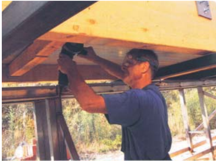
A sample is taken of the roofing.
