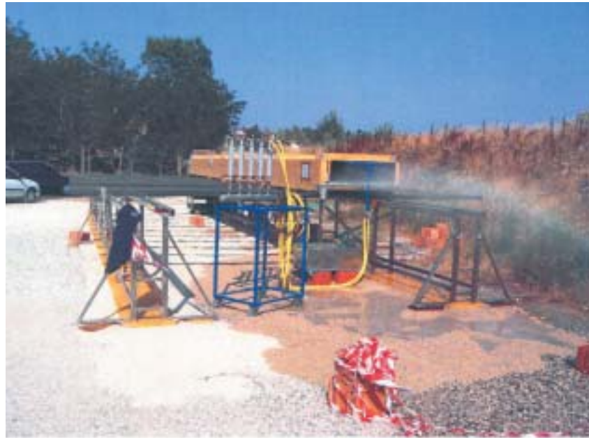
Open side of the tunnel.
