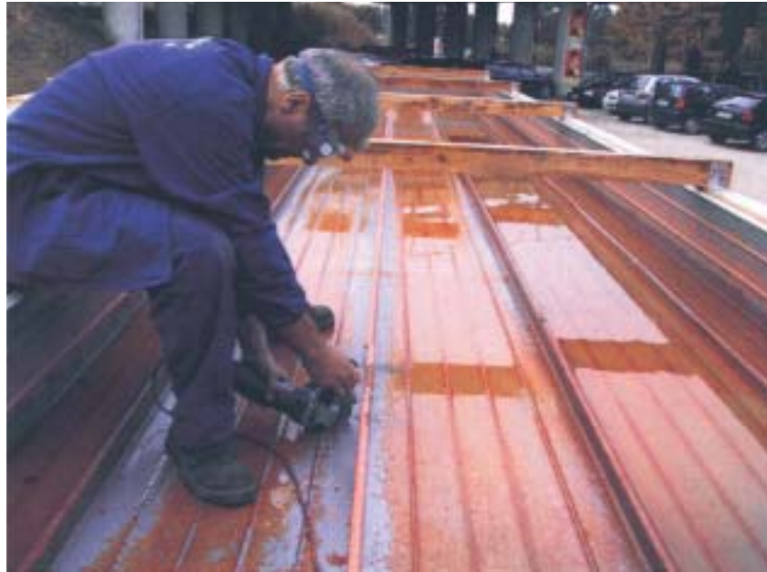
A sample is taken of the roofing.
