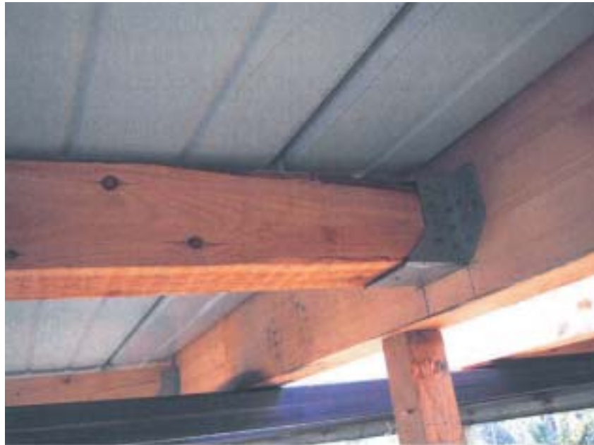
Photograph of the sample subjected to the test: Detail of the connection between the lower cross-members and longitudinal beams.
