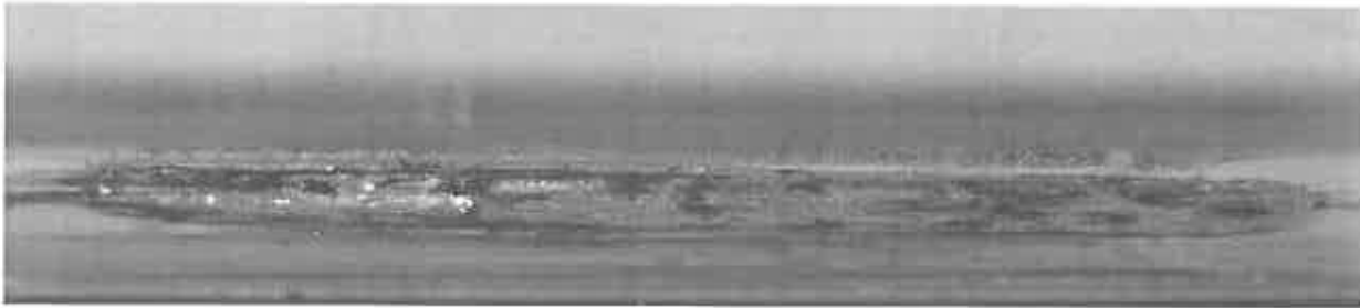
Figure 2.1: Wear and tear zone of the bottom standing seam profile at the central halter after test
